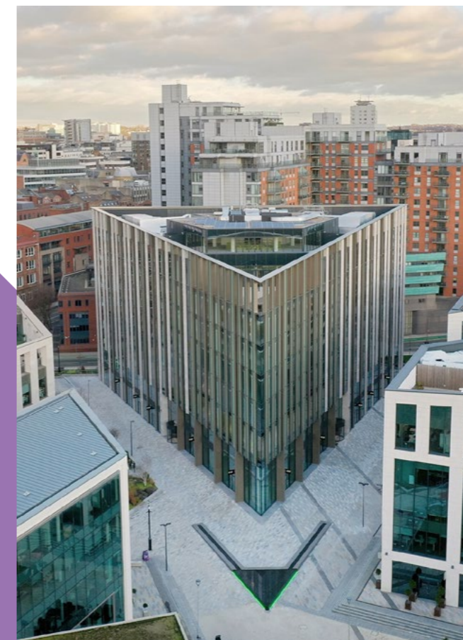
Wellington Place, Leeds
